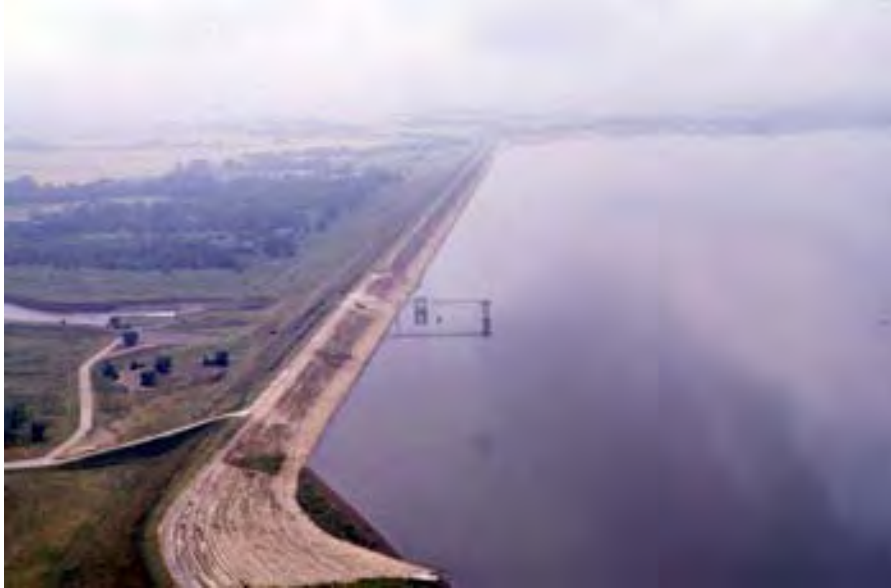
Figure 1. Cheney Reservoir dam, view from north end of reservoir (Photo by USBR).
