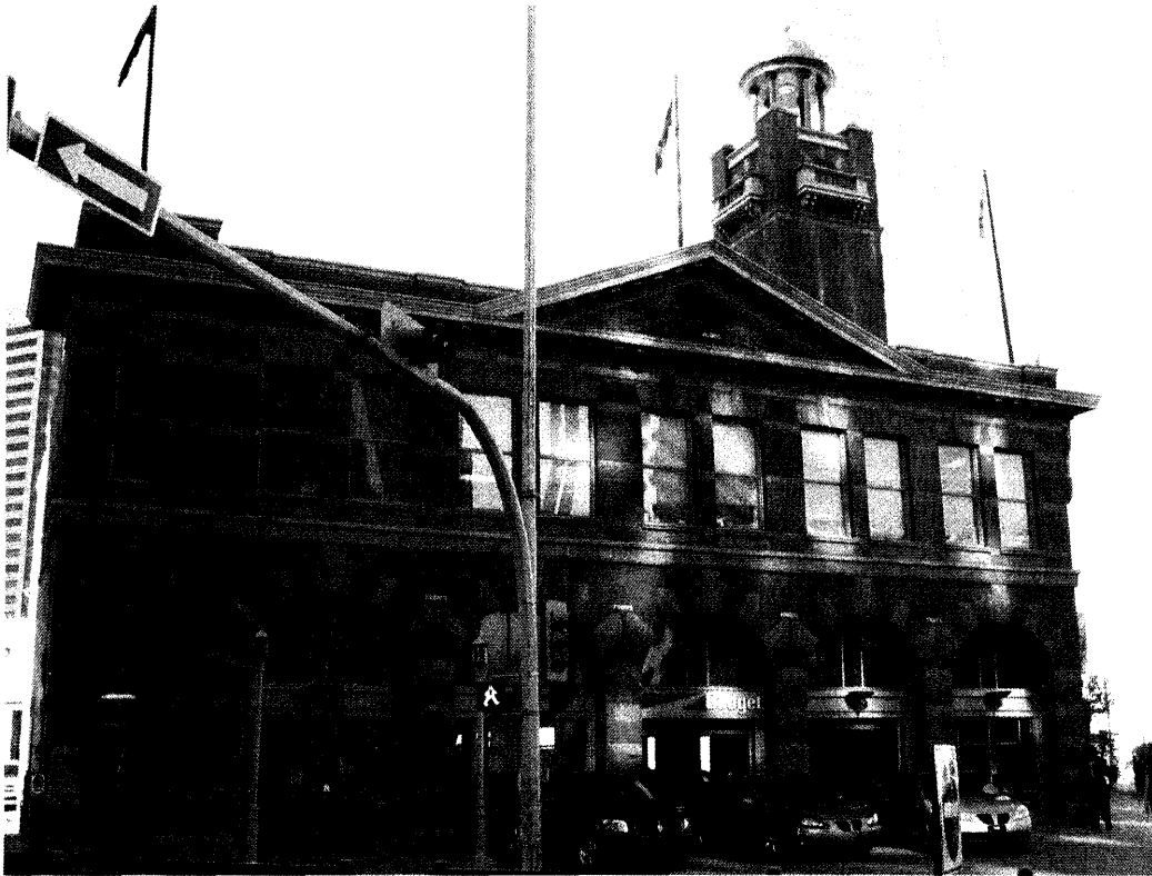
Photo #1.1: South-East façade
