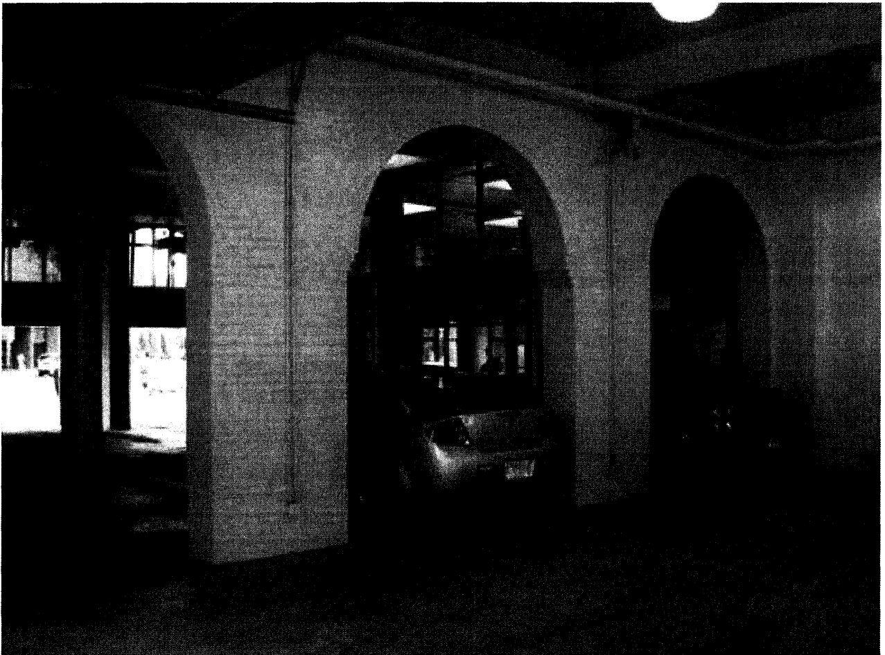
Photo #5.1: The semi-circular arches and brick walls
